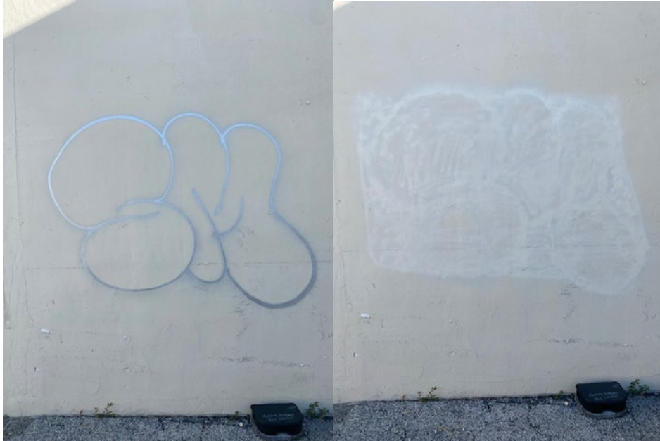
Deputy Westerland cleaned up graffiti behind Kmart.
