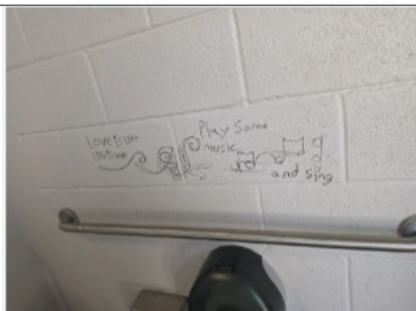
Clean up of Graffiti of the Quay's bathroom.
