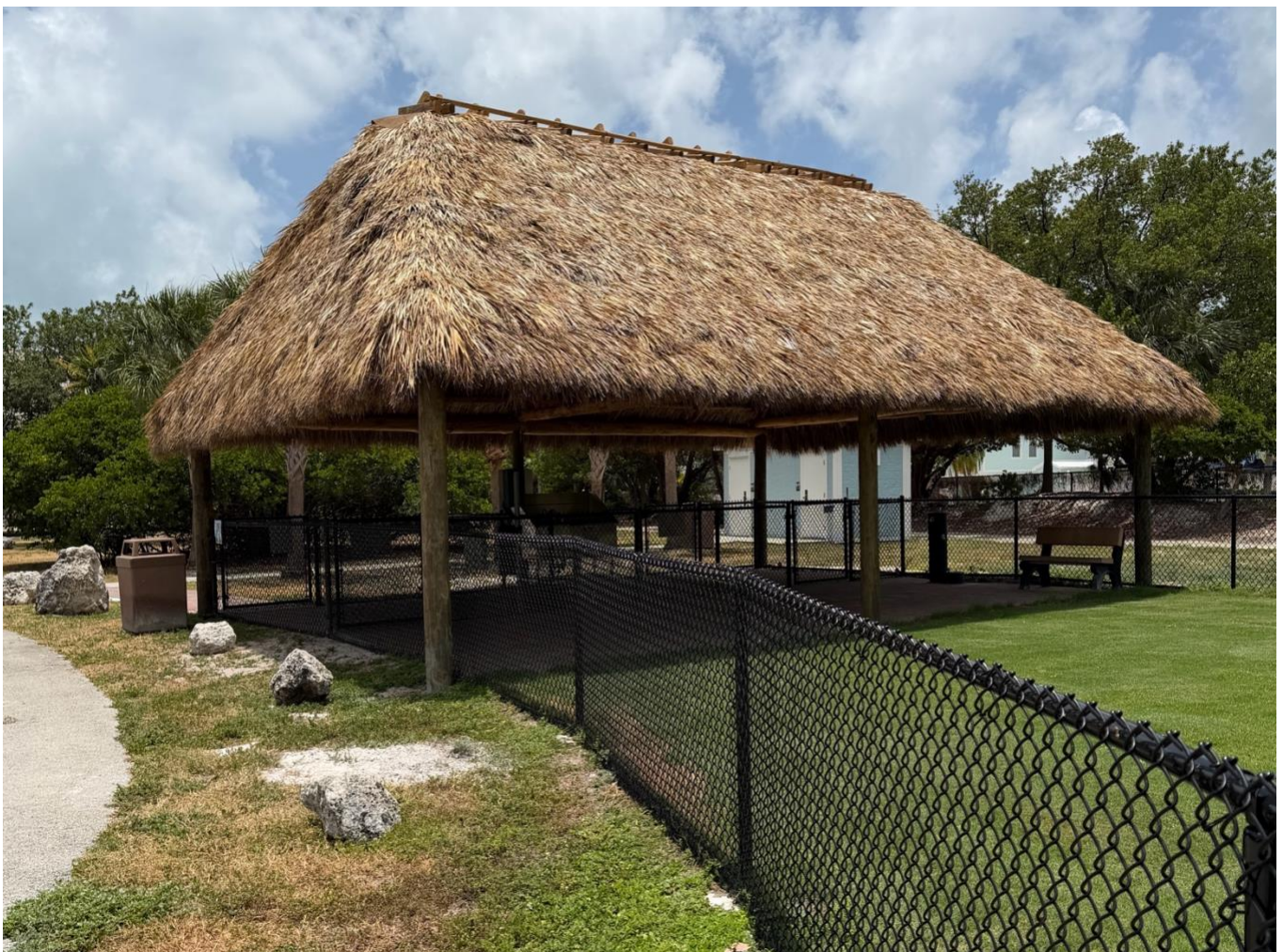
The new tiki shelter at the dog park will provide shade for pets and their owners.
