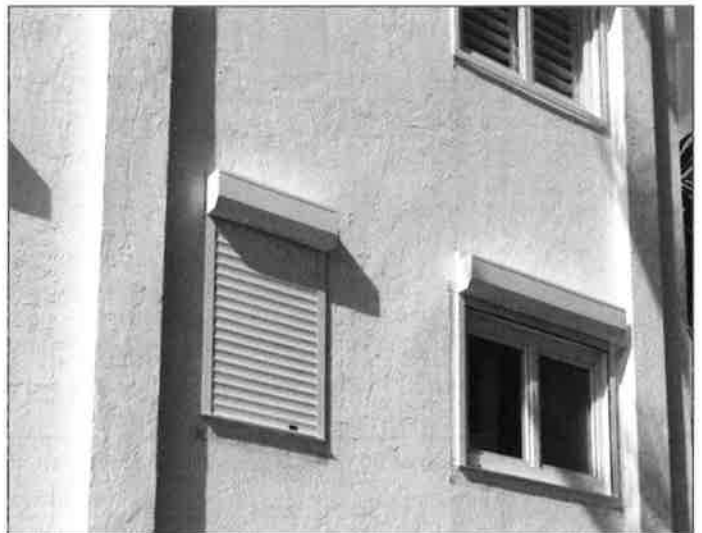
Wind protection measures observed during 2015 site visit.
