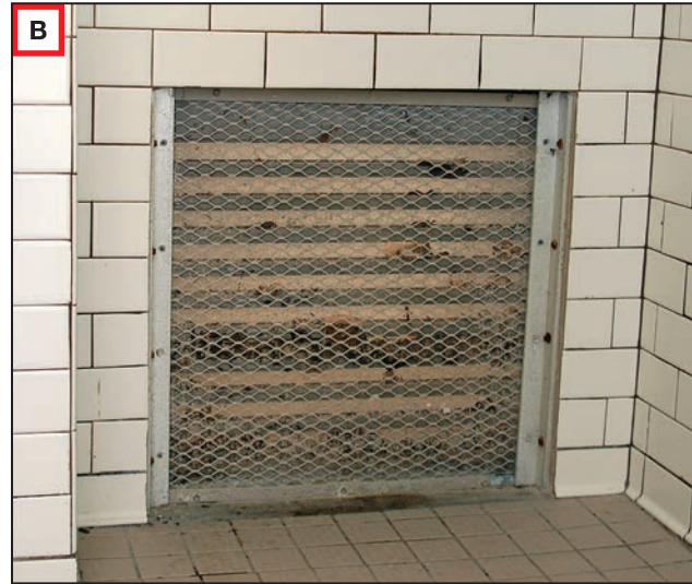
[A] Restroom at Tigertail Beach, Marco Island. The estimated flood depth was 1 to 2 feet, and stormwater and surge from Hurricane Irma carried enough velocity to drive parking lot gravel around the restroom. [B] Flood debris in a vent
