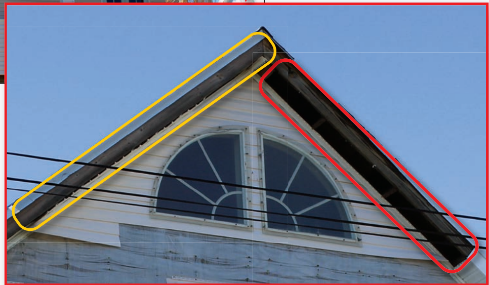
Figure 4-19: House with vinyl soffit damage not caused by fascia loss (EWS = 113 mph; EDWS = 180 mph) (Sugarloaf Key)
