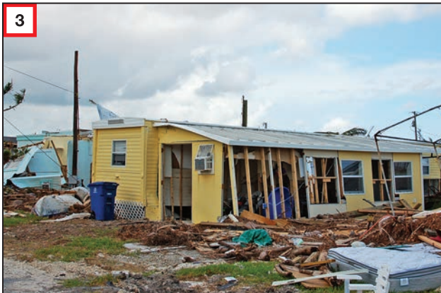
3 Inundation, water velocity, and debris damage to buildings situated farther from the shoreline.
