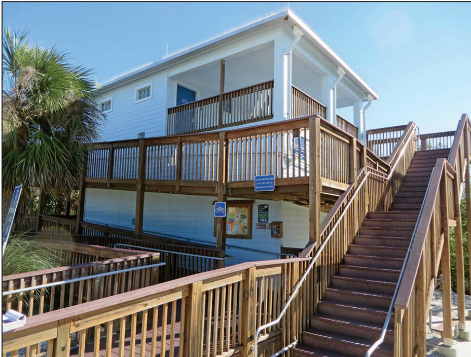
Figure 3-33: Elevated restrooms with ground-level enclosure. Bunche Beach Preserve restroom (Site 1; Lee County), where the degree of flooding in the enclosure, if any, would have been shallow.
