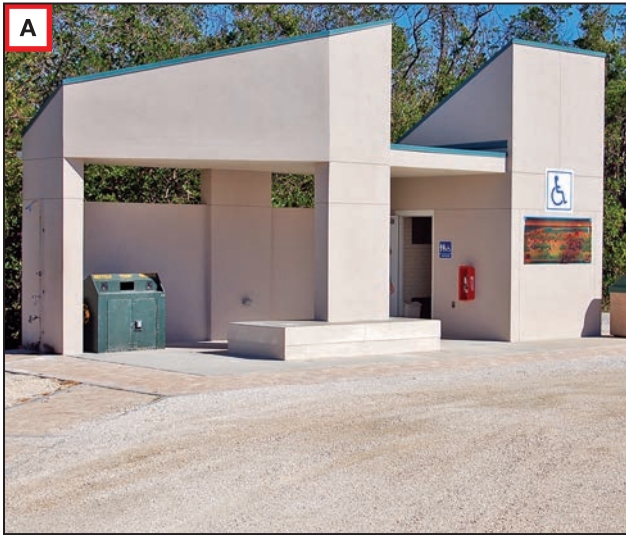
[A] Restroom at Tigertail Beach, Marco Island. The estimated flood depth was 1 to 2 feet, and stormwater and surge from Hurricane Irma carried enough velocity to drive parking lot gravel around the restroom. [B] Flood debris in a vent
