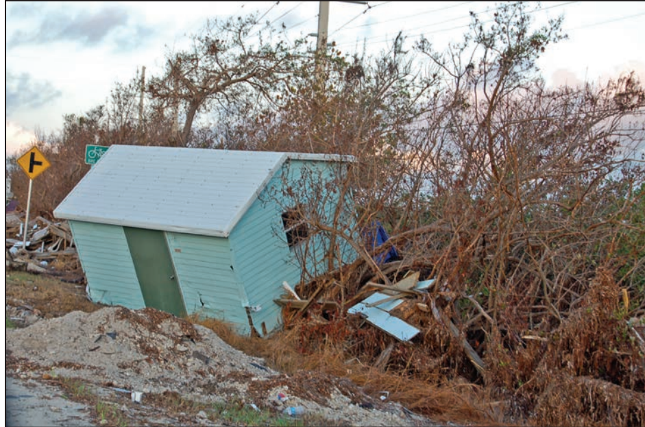
Figure 3-13: Shed that washed across Highway US 1 (Grassy Key, FL)
