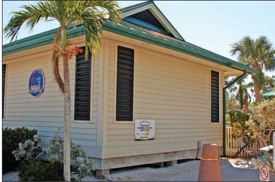
Figure 3-37: Elevated restroom at Tigertail Beach Park (Site 5; Marco Island, Collier County)
