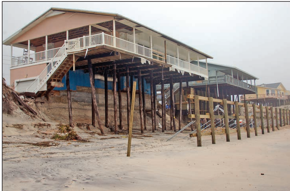
Figure 3-19: Undermined houses constructed on top of the dune (Vilano Beach, FL)
