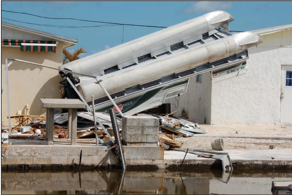
Figure 3-11: Boat and small debris that washed across a canal and onto houses (Big Pine Key, FL)
