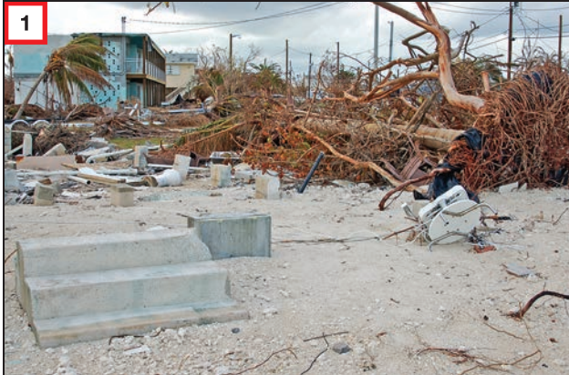
1 House near shoreline and subject to wave action/ high water velocity was washed off its foundation and destroyed.
