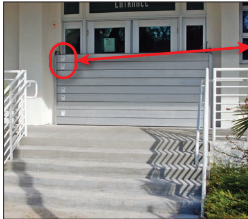
Figure 6: Installed flood panels. Each flood panel has a unique ID number. Also note the tightener bracket at top.
