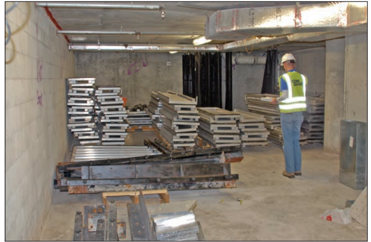
Figure 5: Enclosed storage space for multiple flood panels, stanchions, and hardware
