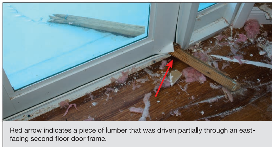
Figure 4-34: Wind-borne driven missile damaged second floor door at the same house as shown in Figure 4-33 (EWS = 114 mph; EDWS = 180 mph) (Little Torch Key)
