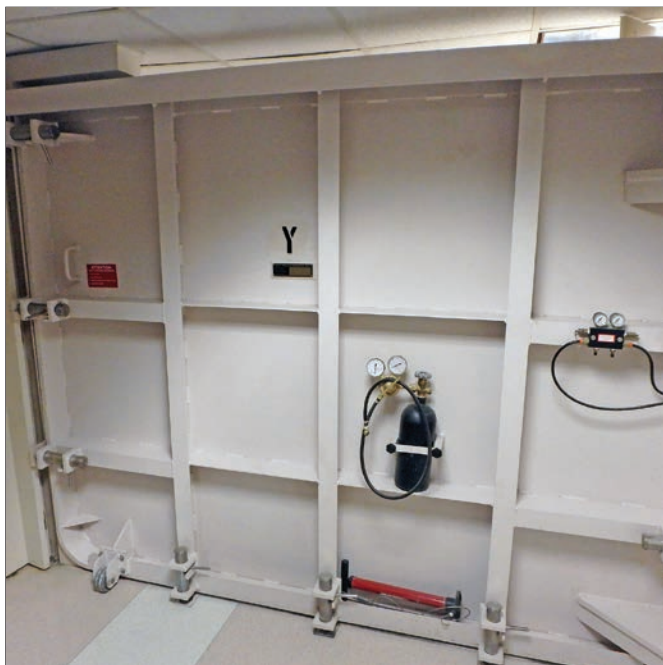
Figure 6: Installed flood panels. Each flood panel has a unique ID number. Also note the tightener bracket at top.
