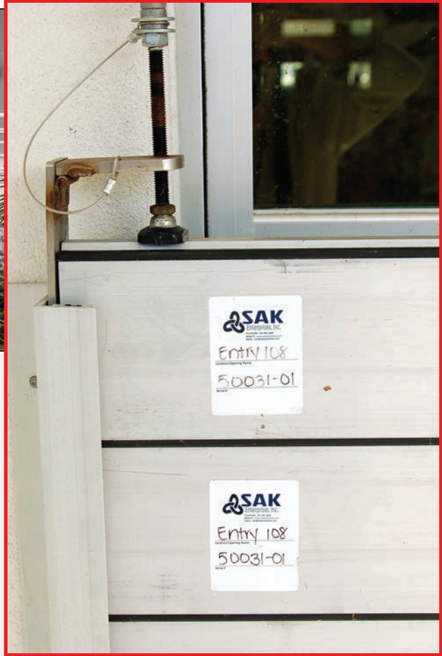
Figure 3-30: Flood plank system deployed at utility company building (Key West, FL)
