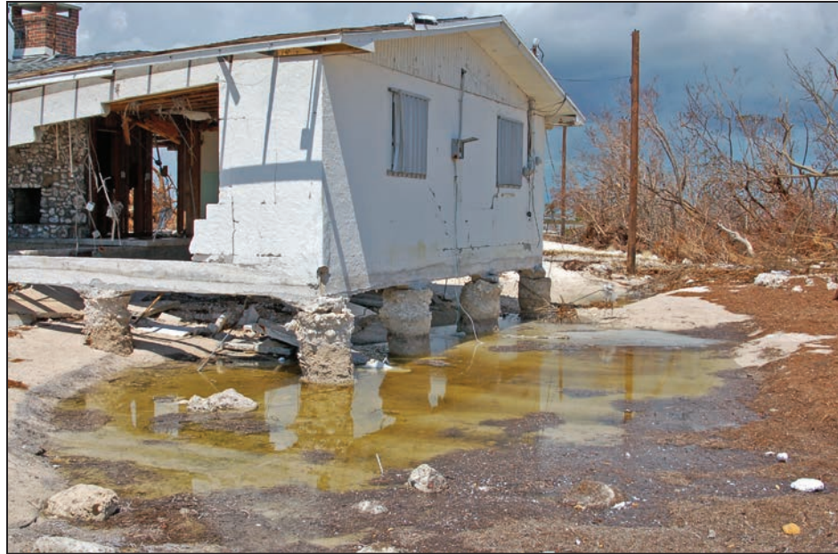
Figure 3-15: Scour was likely due to waves and high-velocity flow at this house on Long Beach Drive (same house is shown in Figure 3-6) (Big Pine Key, FL)
