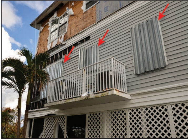
Shutters are shown in place over first-floor glazed openings (red arrows).
