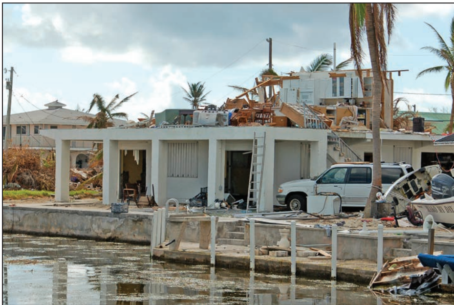
Figure 3-12: Car and debris that washed into a house (Big Pine Key, FL)
