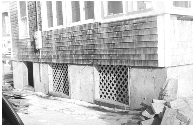
Figure 5-10: Building elevated on crawlspace with openings.
